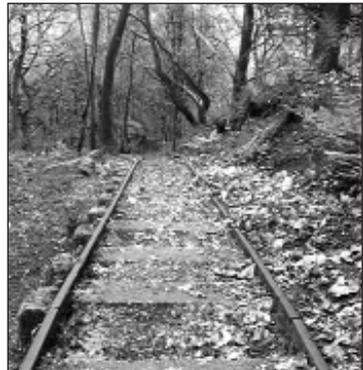
Remains of the narrow gauge railway running from Bulkeley Hill to Peckforton Water Works. Wagons were attached to cables and hauled up the incline by a winding engine.
